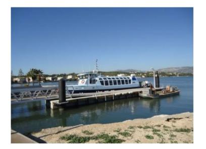
Marine's Bellingham experience in dock construction is unsurpassed. At locations where near shore moorage for cruise ships is not feasible, tender docks can provide the infrastructure needed for cruise lines to access small, local ports. Depending on the site conditions and size of tenders, docks from can range lightweight timber systems to concrete dock systems.
